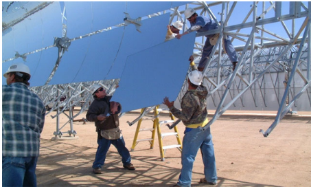
Figure 8. Andasol – a “100 MW” solar power station under construction in Spain. Excess thermal energy produced during the day will be stored in liquid salt tanks for up to seven hours, allowing a continuous and stable supply of electric power to the grid. The power per unit land area will be 10 W/m 2 . Photo: IEA SolarPACES.
